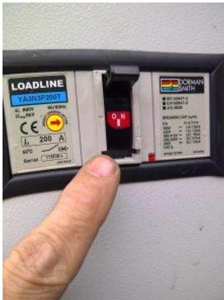
7. When the OFF Load test in Complete Turn the Breaker on the Generator back to ON position
